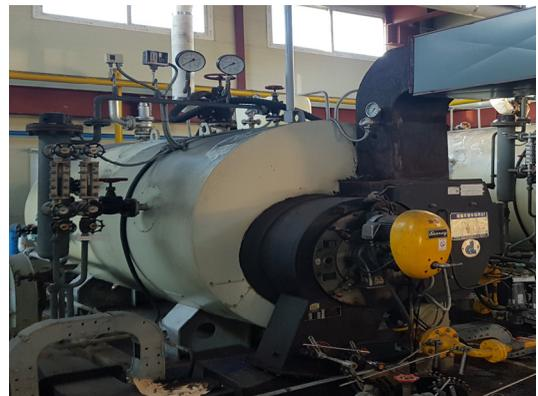
Fig. 1 Photo of a 1.5 ton boiler
