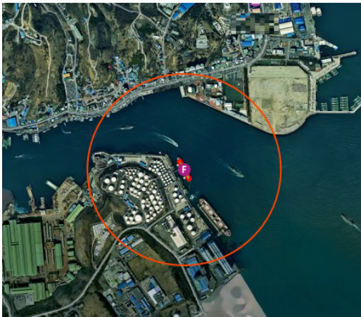
Fig. 4 Leak time 1 min at 220 ppm
