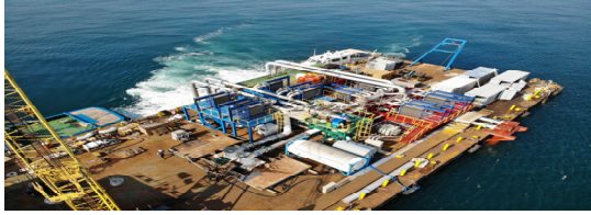
Fig. 1 1 MW OTEC Demonstration plant
